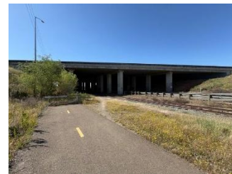
Site of Hwy 50 Under Crossing
