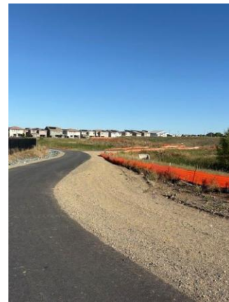
Mangini Ranch Trail under construction
